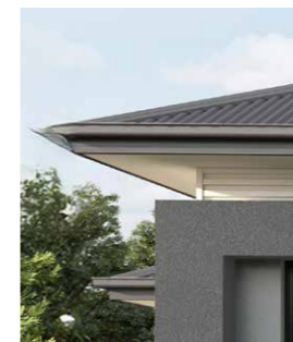
ROOF Hipped roof with clean, closed eaves for a sleek urban profile.
